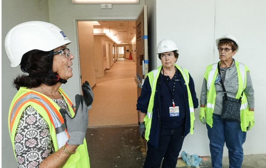
Margaret Fitzwilliam, Director, Capital Renovation Planning & Space Management and winner of the 2020 PFAC Leadership Award, briefs PFA's Sarah Steinberg and Jean Hochron on details of the soon to be completed North Building.
